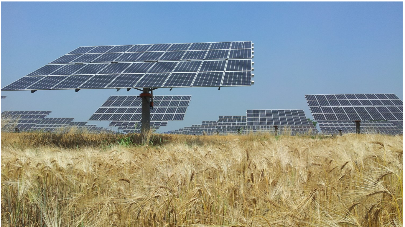
Bifacial agrovoltaic plant at Castelgugliermo.
