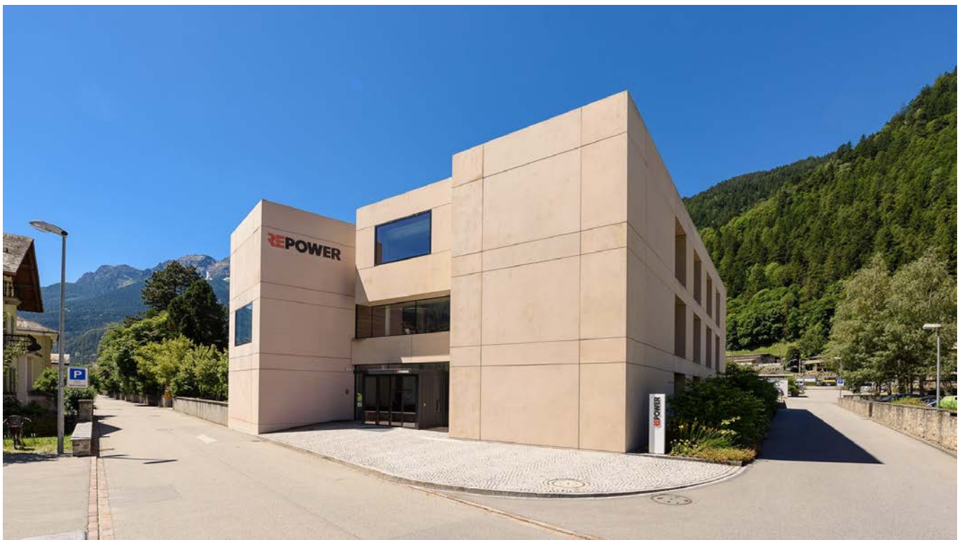
Repower AG headquarters in Poschiavo.
